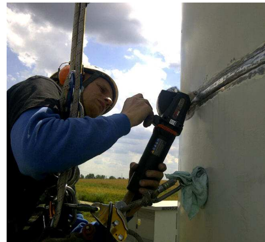
Application of MBX® Bristle Blaster® on wind power station
