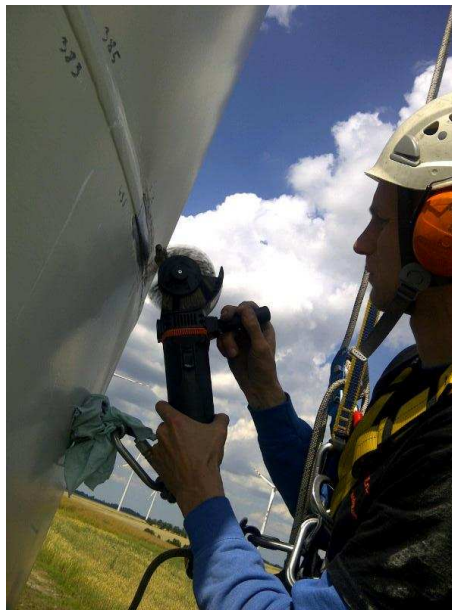
Application of MBX® Bristle Blaster® on wind power station
