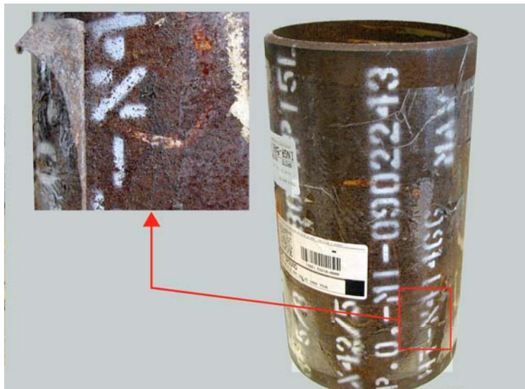
Figure 15 Section of 150mm [6 in] diameter corroded API 5L pipe used for evaluating performance of bristle blasting tool.
